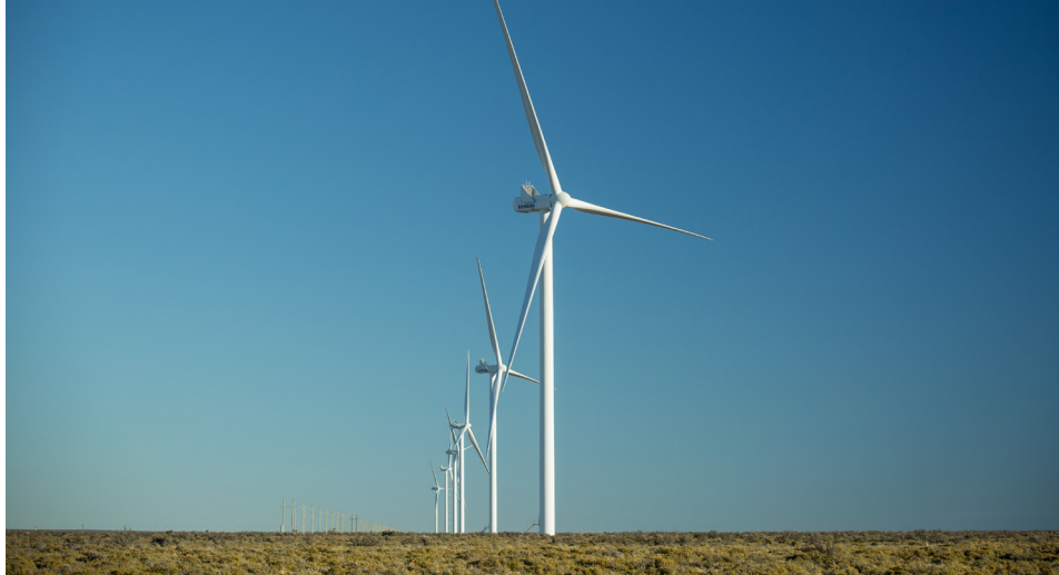
Garayalde Wind Farm, 24 MW, Chubut Photo: courtesy of the Ministry of Energy.
